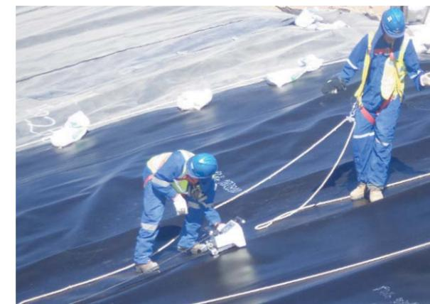
Even uphill to the extreme, the HÜRNER wedge welder HWW 1000 does not face any problems and keeps a consistent speed of movement. Forward movement and optimum heating wedge temperature will be kept, no matter what slope the device rolls up.
